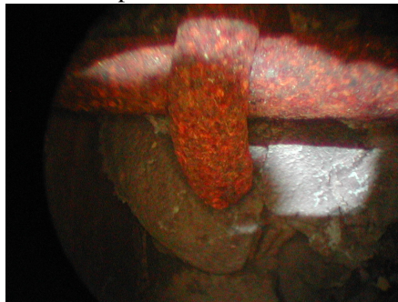
J-bolt and pin intersection.
