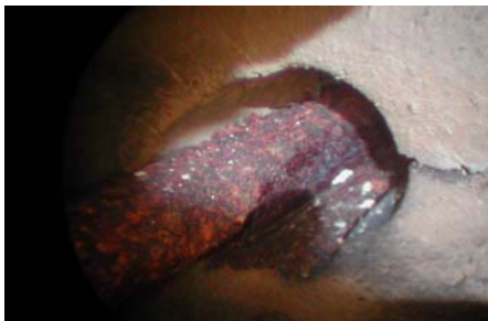
Cracked rib.
